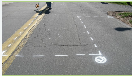
Typical survey paint markings
