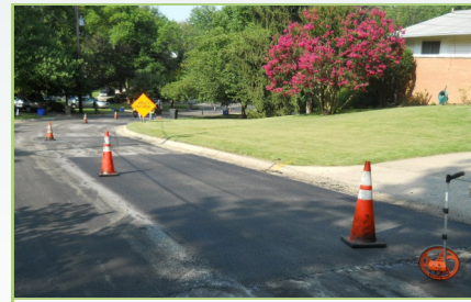
New patch is flush with existing pavement
